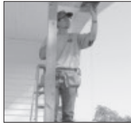
6. Using a plumb tool, find and mark bottom position on floor.
