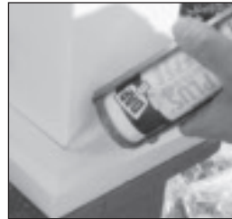
12. Slide skirt into position and caulk seam.
