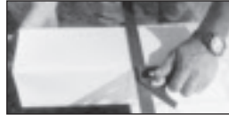
3. If using handrail, check local building codes for minimum rail height. Decide how much is to be trimmed from each end of PermaPost. Top and bottom mounting plates are 1/8" thick. Mark post 1/4" shorter than total opening.
