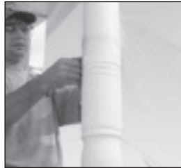
10. Check post for level and remove temporary support.
